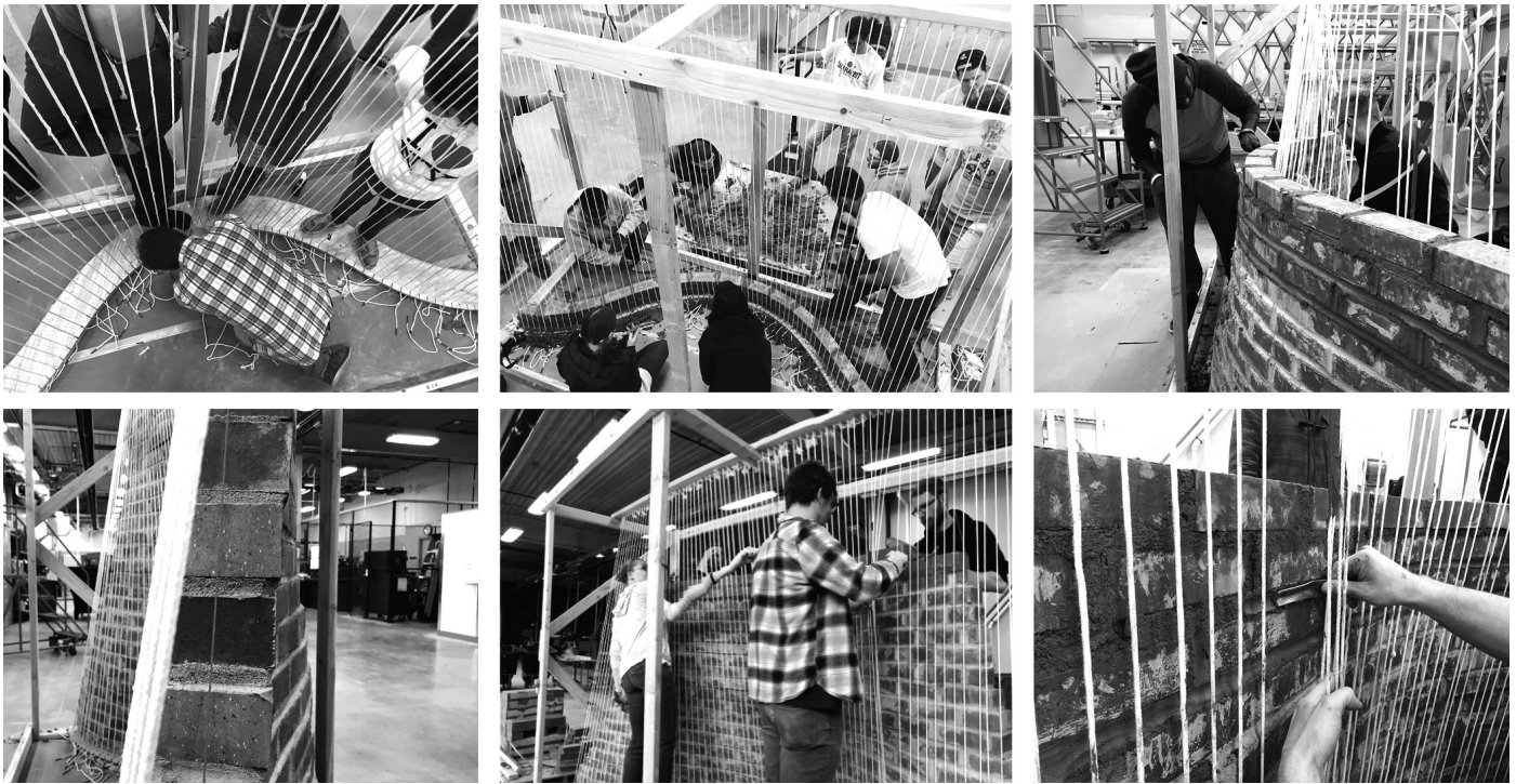
Figure 3: Ruled surface brick wall construction, Curved Walls: Eladio Dieste and Ruled Surfaces Workshop, South Dakota State University.
